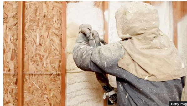
Spray foam insulation is applied with a spray gun and expands to fill a given area, setting to form an insulation layer
