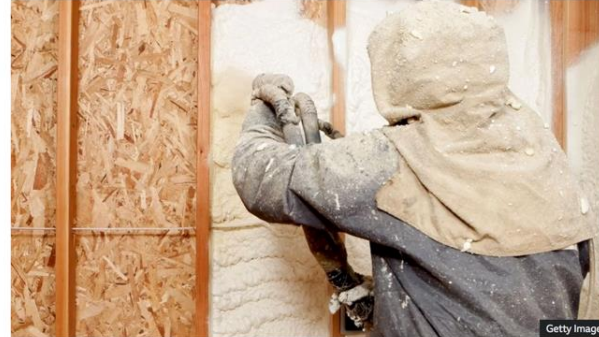
Spray foam insulation is applied with a spray gun and expands to fill a given area, setting to form an insulation layer
